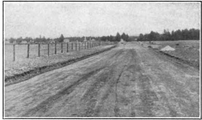
Straightaway on Tacoma course before it was ironed out
